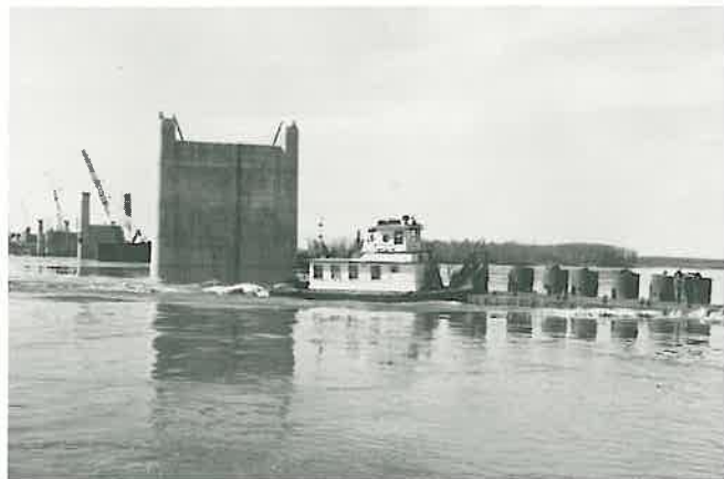
"Buckets" of concrete are barged out to a pier under construction.
